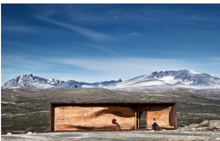
Project Name Tverrfjellhytta - Norwegian Wild Reindeer Centre Pavilion Photographer Ketil Jacobsen Copyright holder © Ketil Jacobsen
